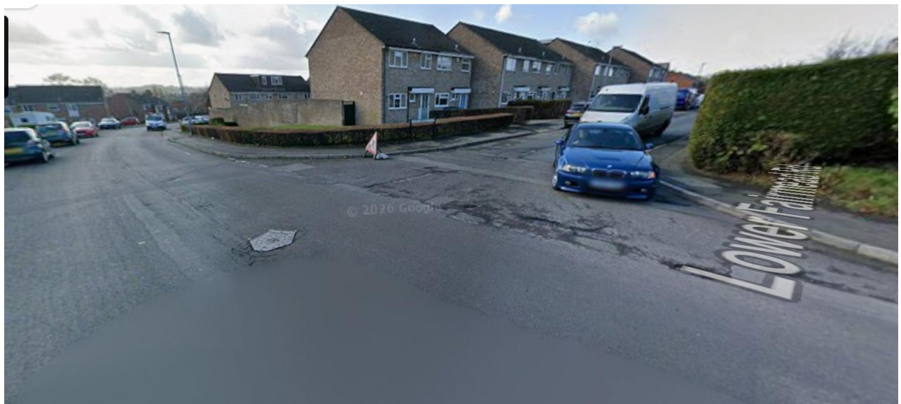
Lower Fairmead Rd – current road markings and condition
